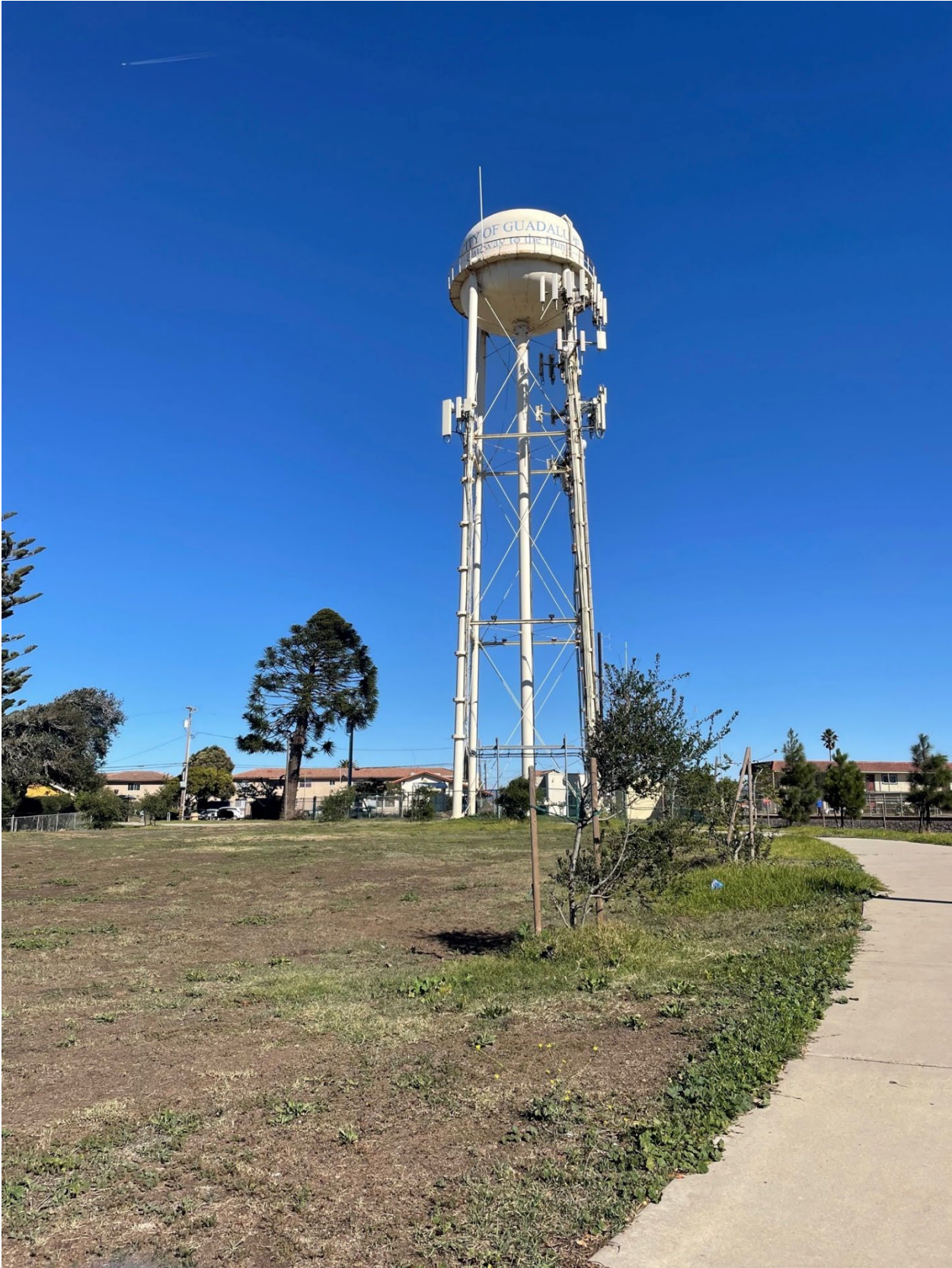
Elevated Tank – View from South
