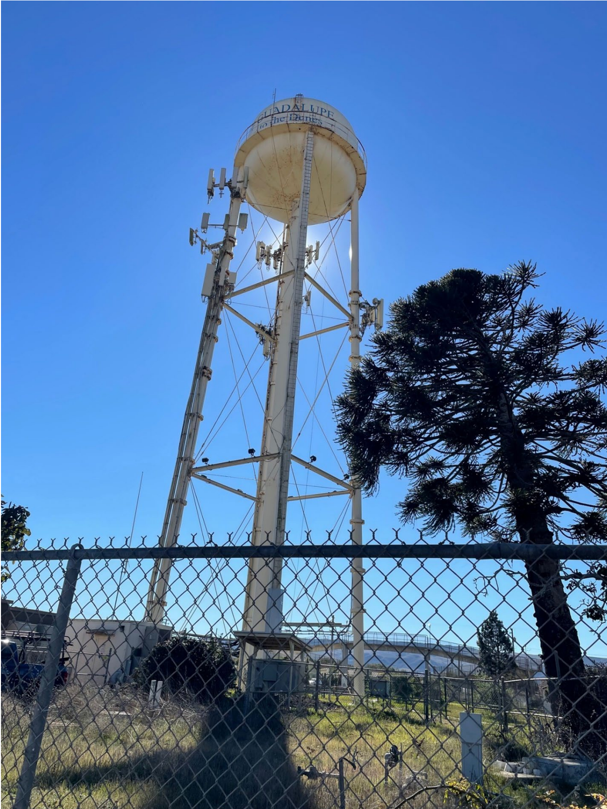
Elevated Tank – View from North
