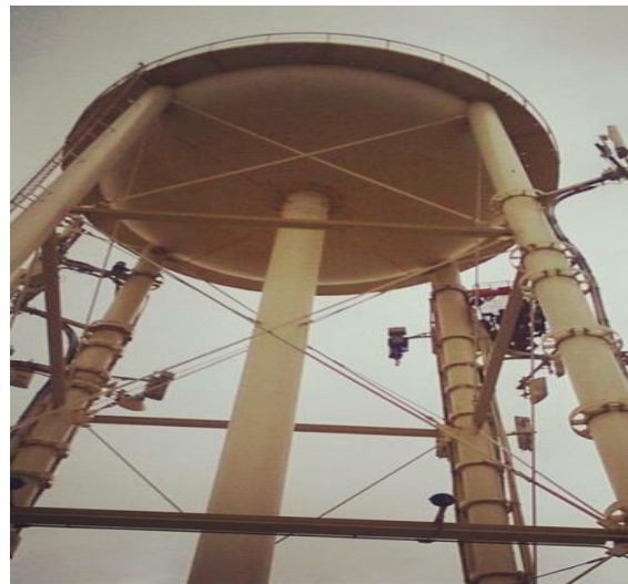
City of Guadalupe Elevated Water Tank
