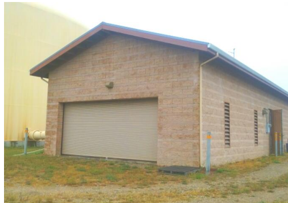
City of Guadalupe Obispo Boosting Station
